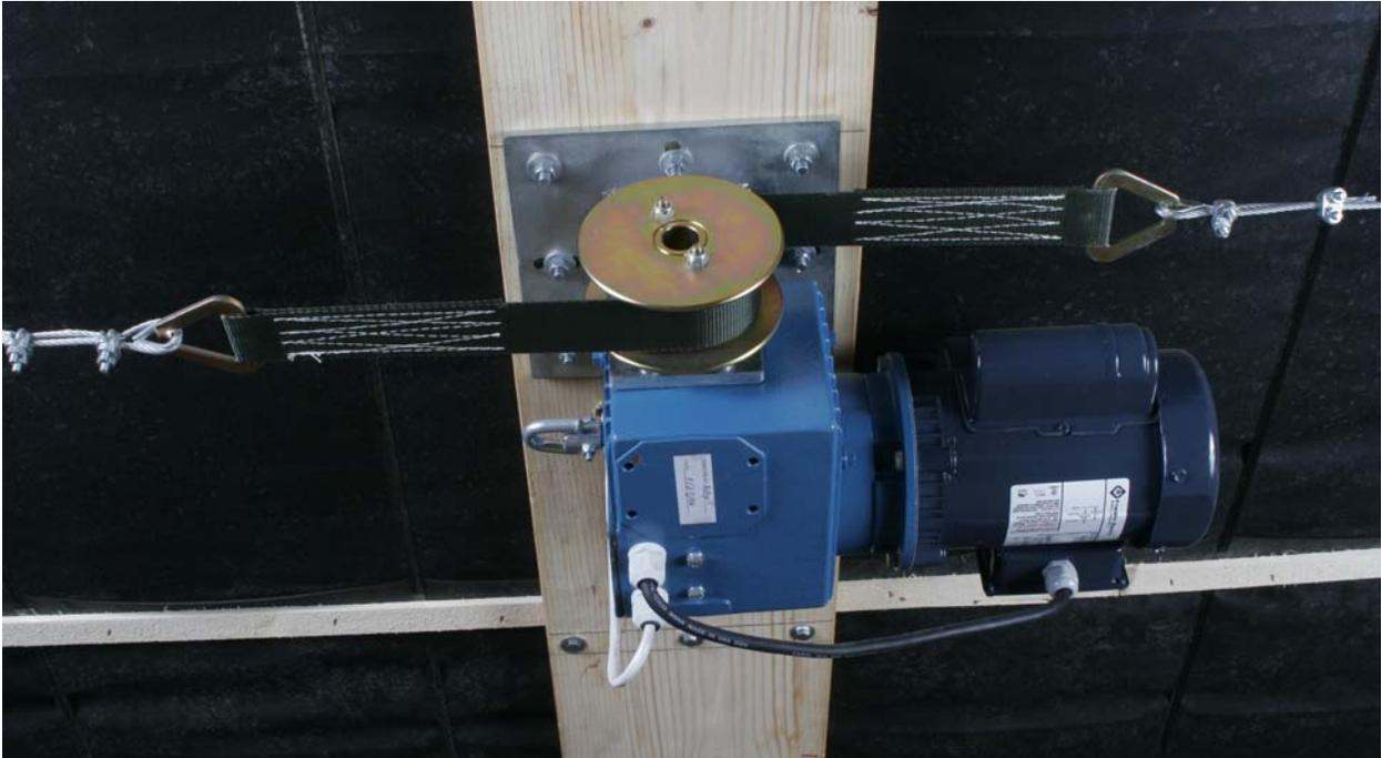
1. Using the cardboard template, drill holes in a 2" plank and mount the Curtain/Vent Machine as shown above. Bolt the unit mounting plate to a 2x12 plank (or two 2x6's) that is (are) secured to the house studs or rafters. The machine may be mounted on the plank before the plank is bolted to the wall or ceiling. If the plank is bolted to the wall or ceiling first, there are slots in the base that will slip over the head of a 3/8" lag bolt to hold the machine while it is being secured.
